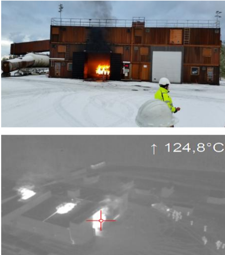
Figure 116. Image outside the firehouse (upper), and FLIR image (below) showing the highest temperature of 124.8 °C near the doorway of the firehouse.
